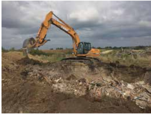
An excavator makes way for prairie restoration at the Bennet Property.
